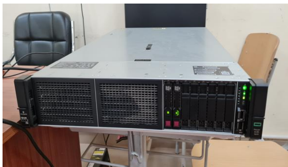
Installation of Server in Simulation and Visualization Laboratory, Department of Atmospheric Science
